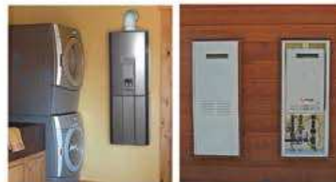
CUSTOM INSTALLATIONS to match the outside appearance of the home or to blend in with the interior (shown with optional pipe cover).
