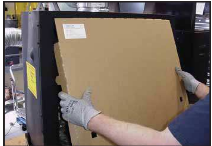
Figure 13.8 Installation of Splatter Guard
