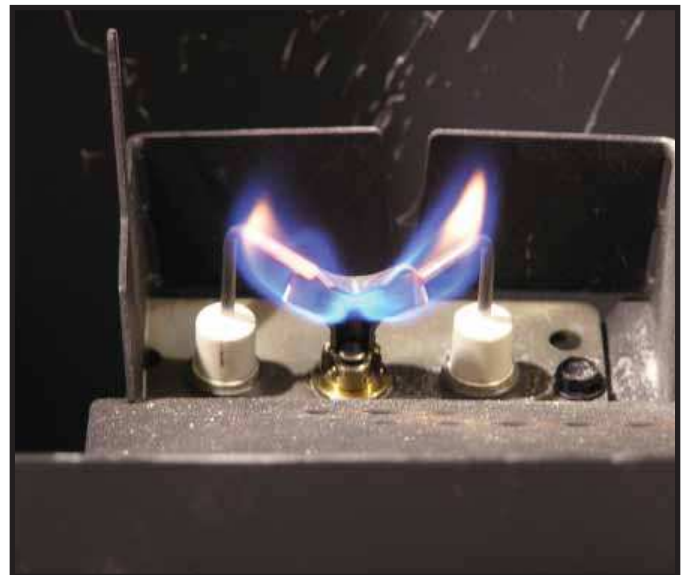
Figure 3.1 IPI Pilot Flame Patterns
