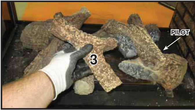
Figure 14.9. Placement of Log #3
