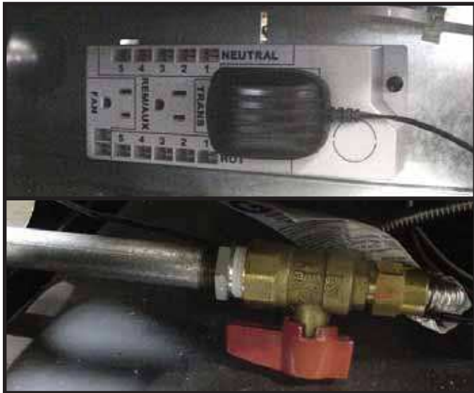
Figure 13.5 Preparation to Install Splatterguard
