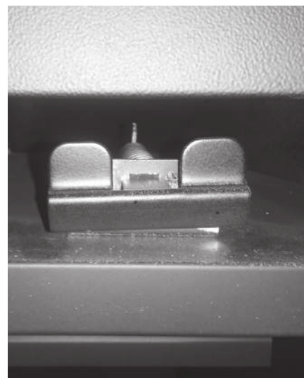
Figure 55a - Glass Frame Latch
