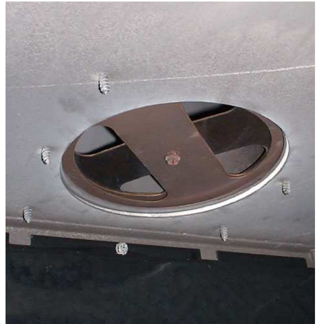
Figure 9 - Restrictor disc (shown with 2 discs closed)
