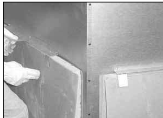
Figure 7.1 Unpacking Back Refractory
