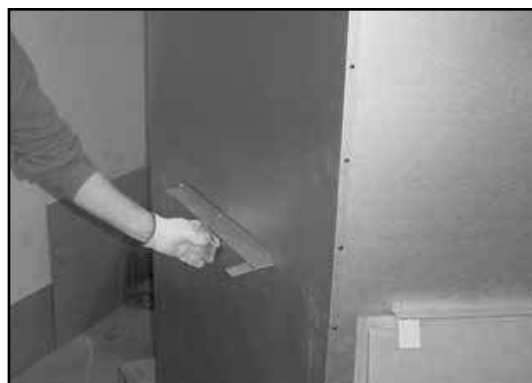
Figure 7.2 Bending Refractory Shipping Tabs Back Down
