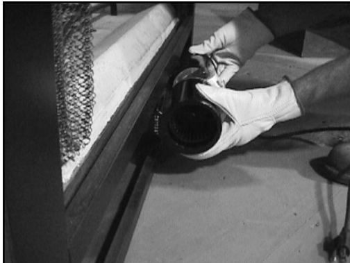
Figure 4 - Inserting the Fan into the Fireplace
