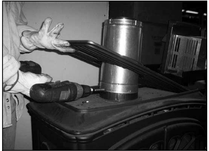
Figure 7 Fasten SLP Vent to Stove
