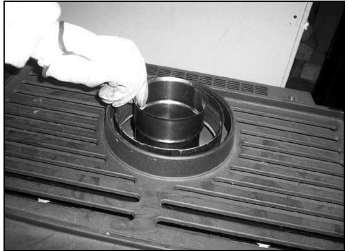
Figure 11 Install SLP-SAM Adapter
