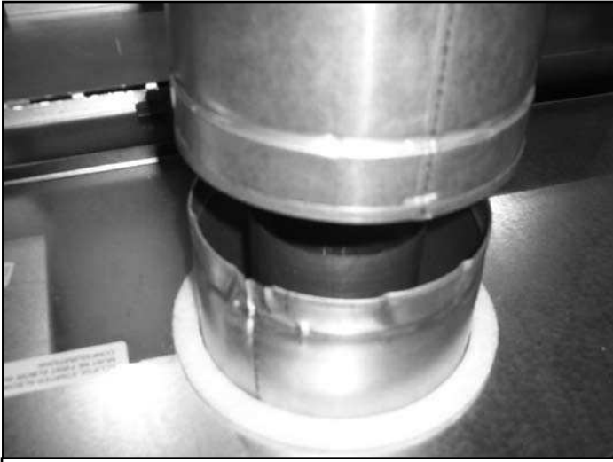
Figure 5 SLP Pipe onto SL-D Collar
