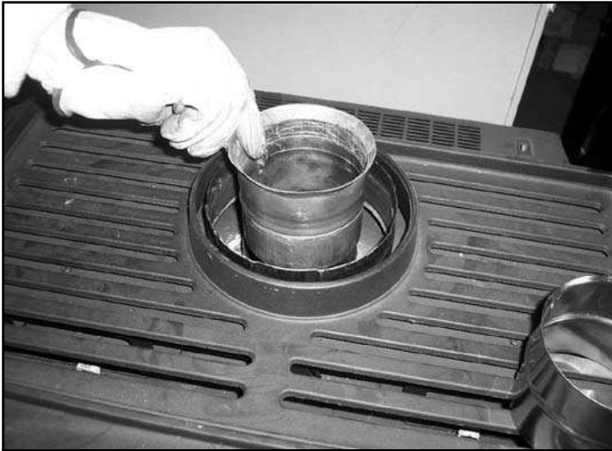
Figure 10 Remove SL-D Adapter
