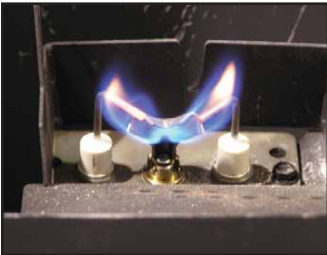
Figure 3.2 IPI Pilot Flame Patterns
