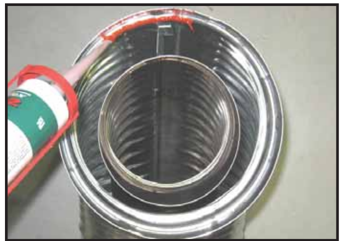
Figure 10.2 High Temperature Silicone Sealant
