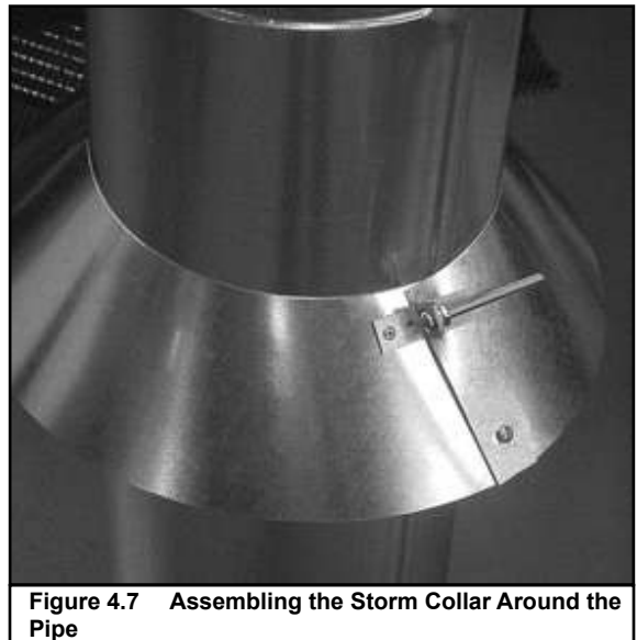
Figure 4.6 Assembling the Storm Collar
