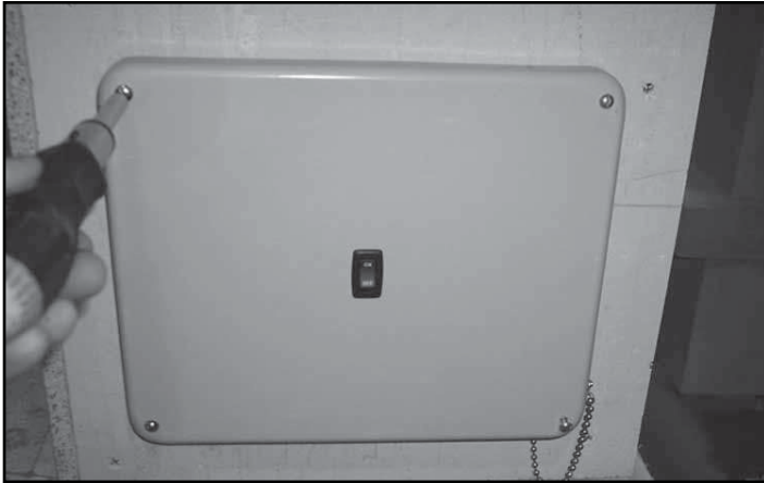
Figure 6.3 Remove Control Cover
